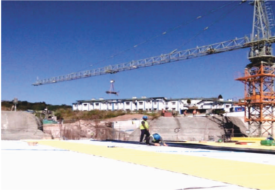
Waterproofing of Underground RCC Structure
