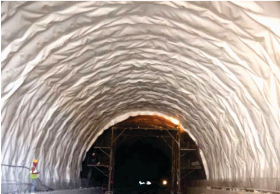
Tunnel Water Proofing with PVC Membrane
