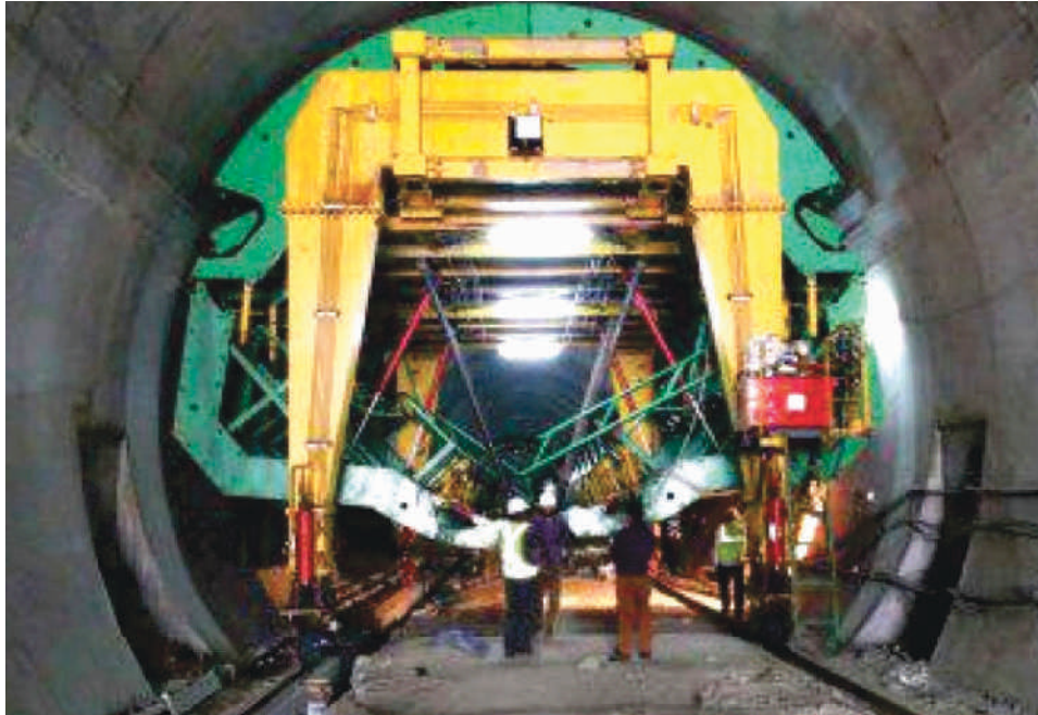
Tunnel Water Proofing with PVC Membrane
