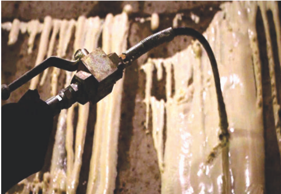
Two Component PU Grouting
