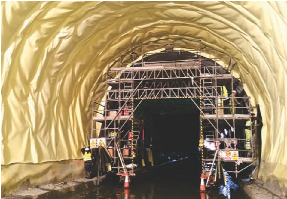
Tunnel Water Proofing with PVC Membrane
