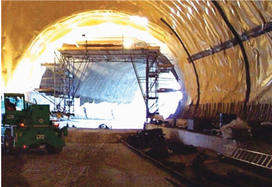
Tunnel Water Proofing with PVC Membrane
