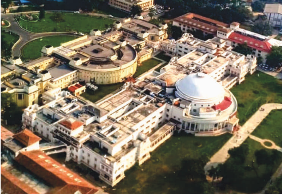
Water Proofing Work for the Newly Constructed Bihar Vidhan Mandal
