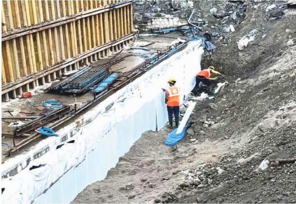
Waterproofing of Underground Structure
