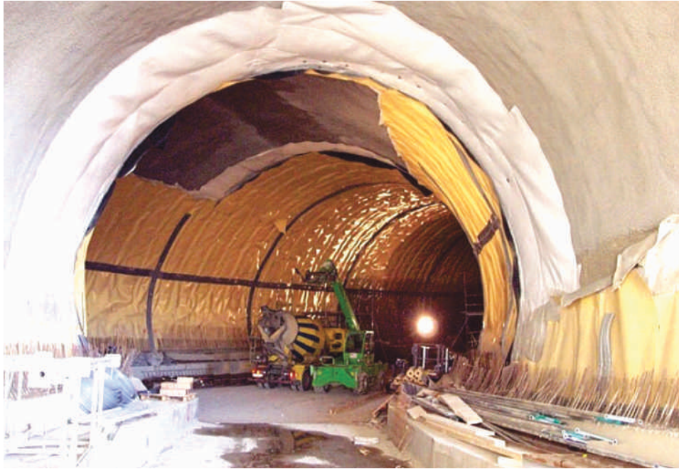
Tunnel Water Proofing with PVC Membrane
