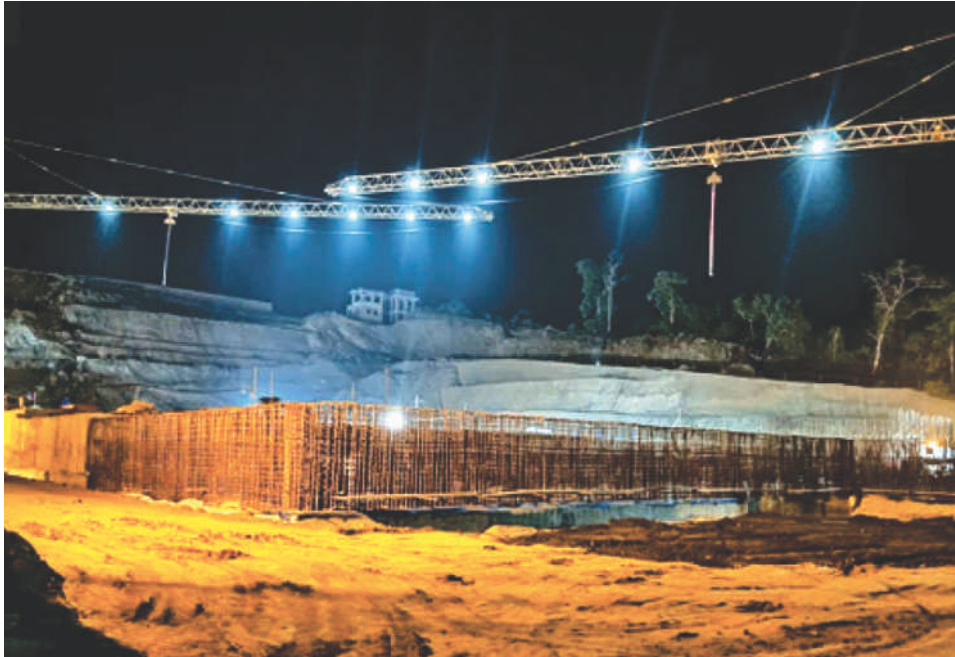
Waterproofing of Underground RCC Structure
