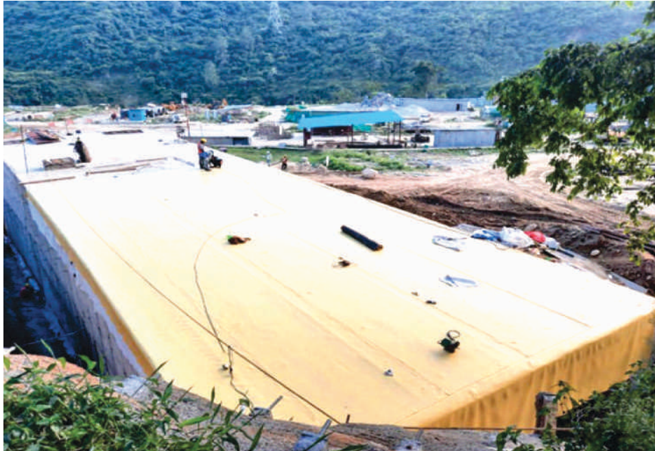
Waterproofing of Underground RCC Structure
