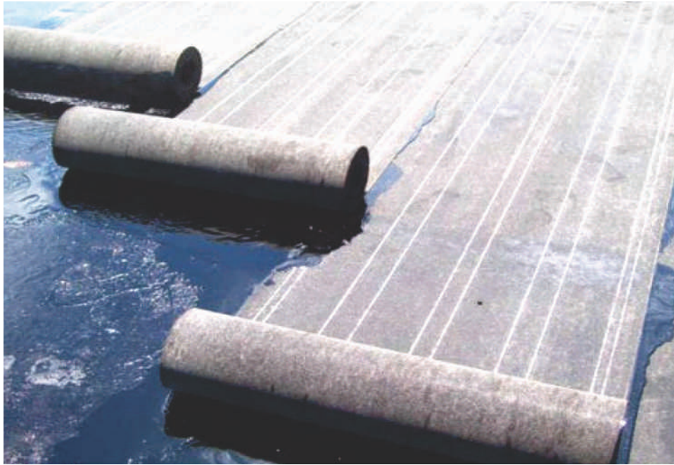
Waterproofing of RCC Shell Roofs of Overhaul
