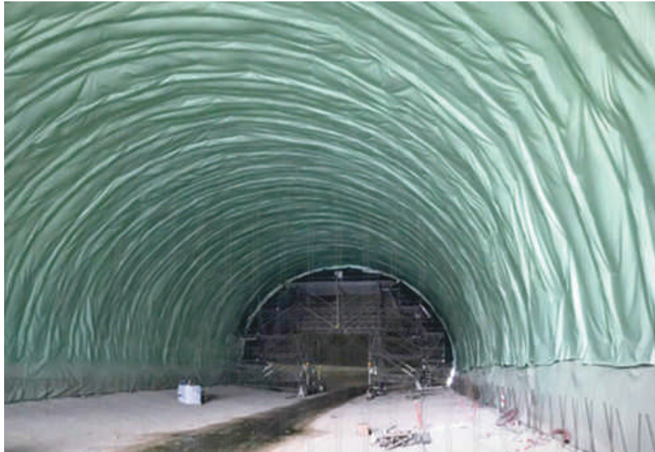
Tunnel Water Proofing with PVC Membrane
