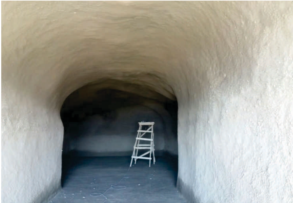
Pressure Release Water Proofing of Cave
