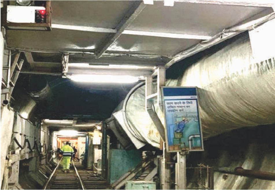
Grouting Work in Hydro Electric Project
