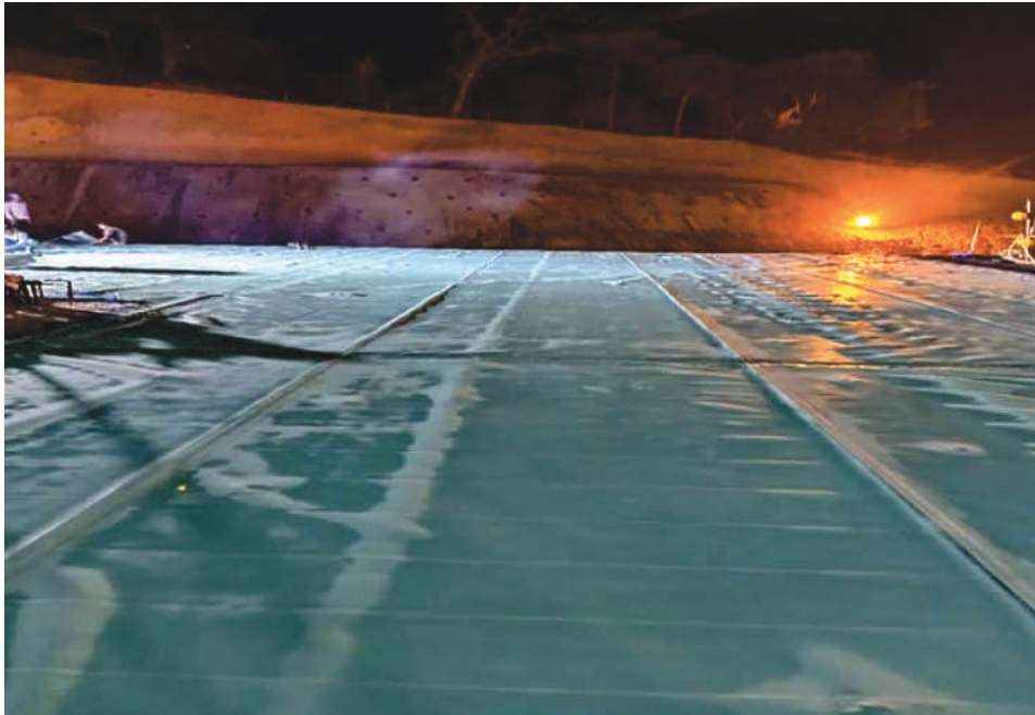
Waterproofing of Underground RCC Structure
