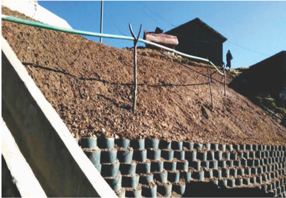
Restoration of Helipad and Construction of Retaining walls with Geoweb Technique
