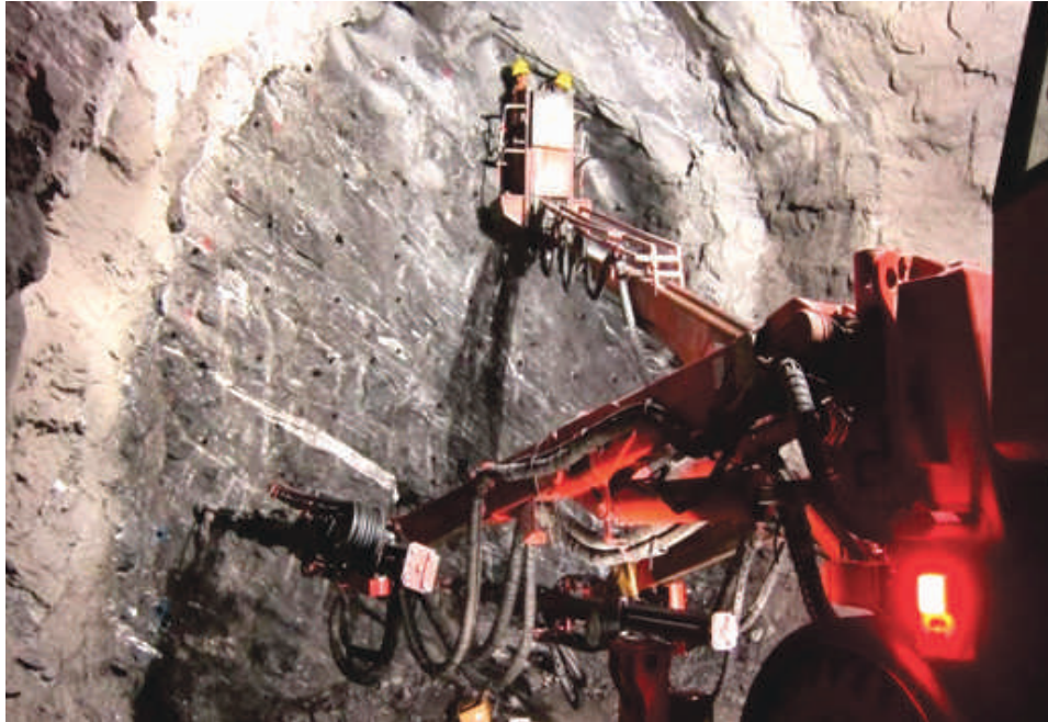
Tunnel Excavation and Rock Support
