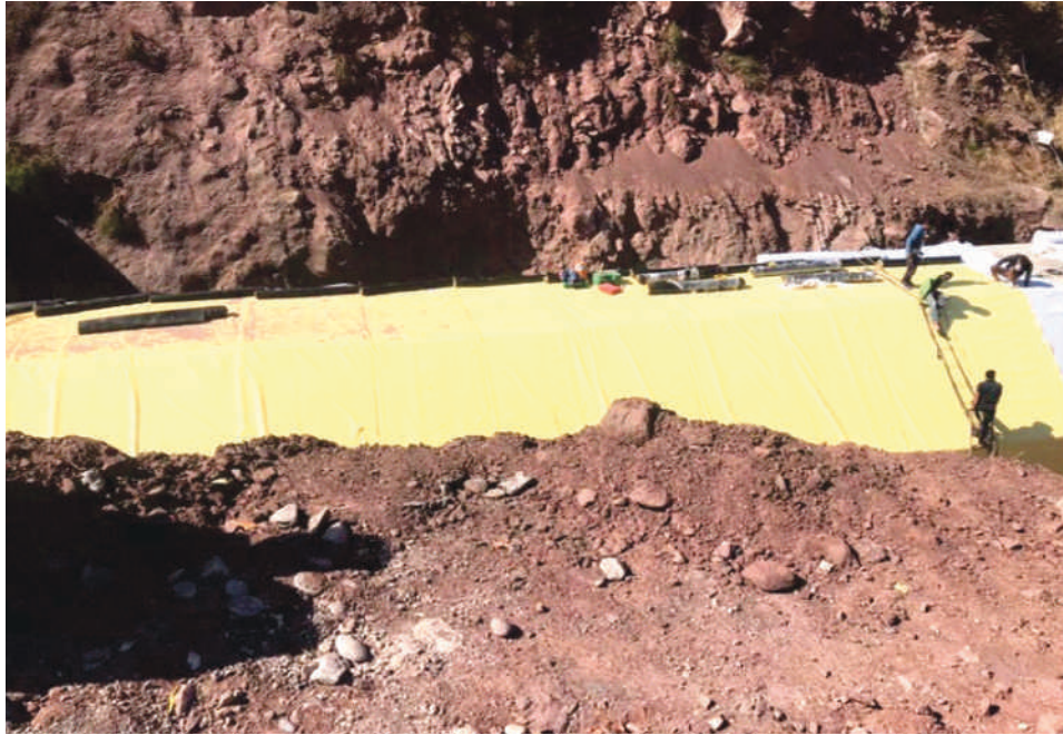
Tunnel Water Proofing with PVC Membrane
