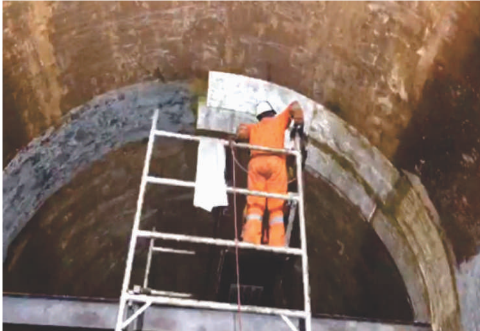
Repair of Ridge Reservoir at Shimla (Himachal Pradesh)
