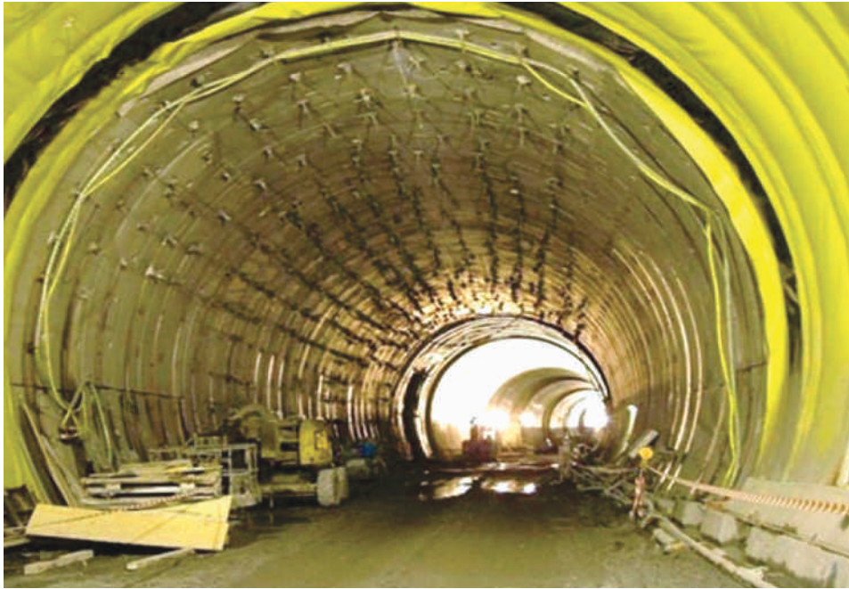
Tunnel Water Proofing with PVC Membrane
