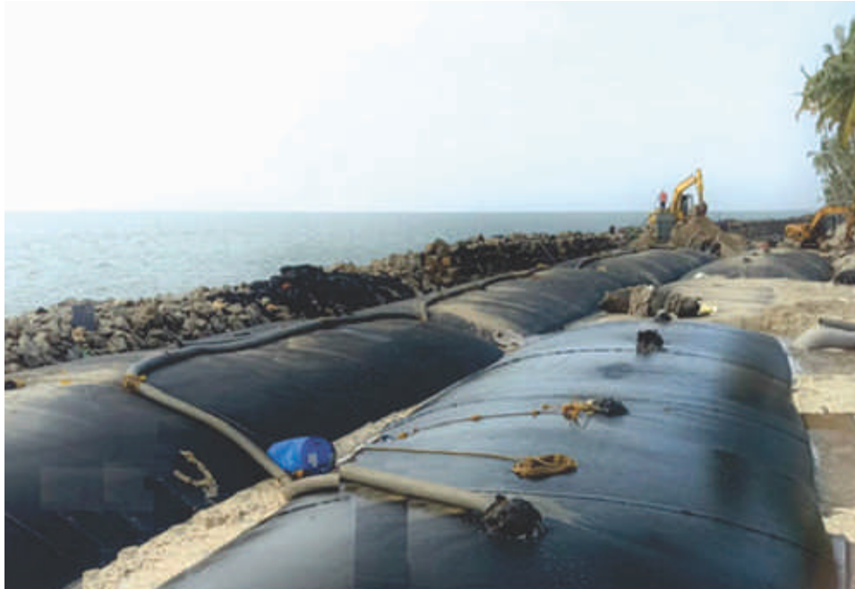
Coastal Protection Work Using Geotubes
